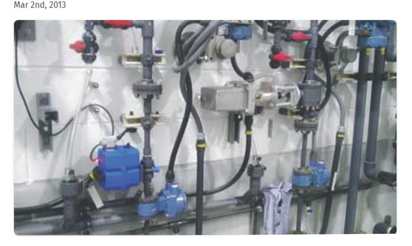
A thermoplastic control valve was compared side by side to a metal control valve and was found to be 80% more accurate than its metal counterpart.
